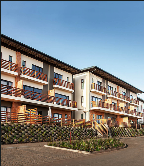
Cotswold Fenns Residential Estate Contract Value: R300 mil. | Description: 186 Contemporary Apartments and Management Office, in Hillcrest.
