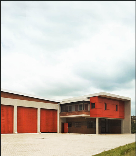
Verulam Fire Station Contract Value: R22 mil. | Description: 1 400m² Fire Station and Emergency Response Unit, in Verulam.
