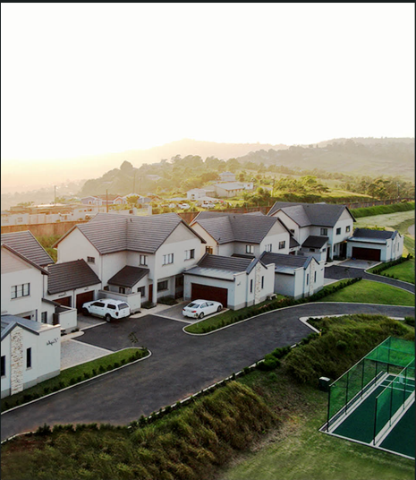
Tewkesbury Terraces Contract Value: R40 mil. | Description: 36 Townhouses, Clubhouse & Park in Cotswold Downs Estate, Hillcrest.
