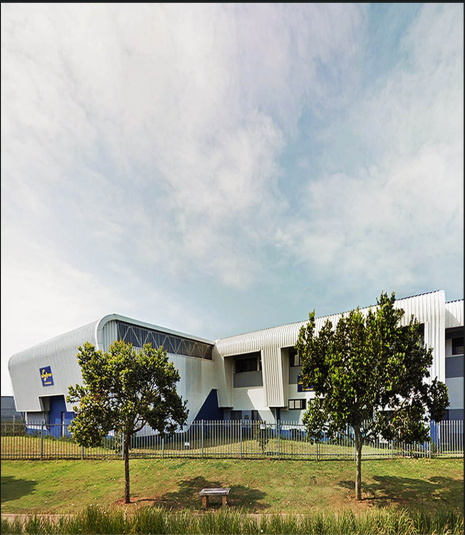
Tren Tyre Fitment Centre Contract Value: R25 mil. | Description: 1 750m² Regional Tyre Fitment Centre, Offices and Storage, in Durban.
