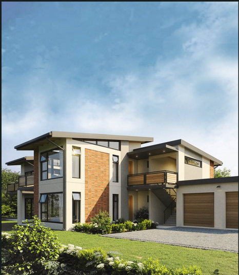
Jacana Eco Estate Contract Value: R70 mil. | Description: 30 Freestanding and Duplex Residential Units, in Hilton.
